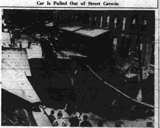
The wreckage of an automobile is hauled out of a 40-foot hole in a West Philadelphia street which caved in after continuous rains flooded a sower.
